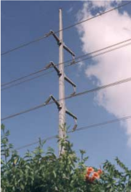
Completed Transmission Line
