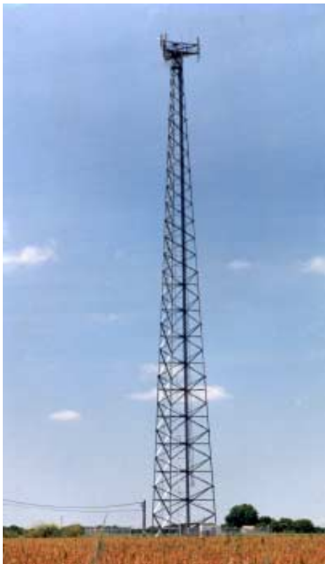
Cellular Tower, McAllen, TX
