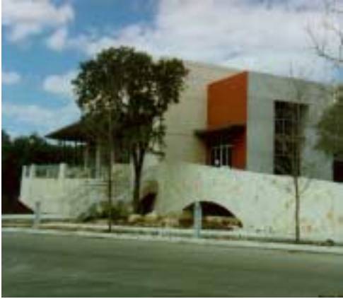
Harris Communications, San Antonio, TX
