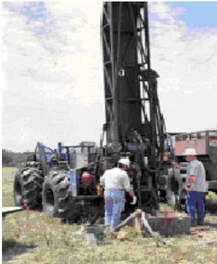
DCE Technicians drilling to recover soil samples for laboratory testing
