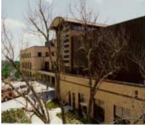
LBJ Student Center and Parking Garage at Southwest Texas State University in San Marcos, TX
