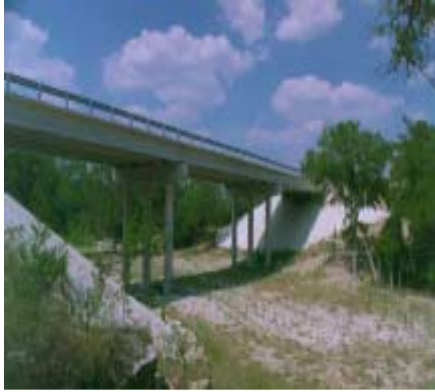
River Mountain Bridge Boerne, TX
