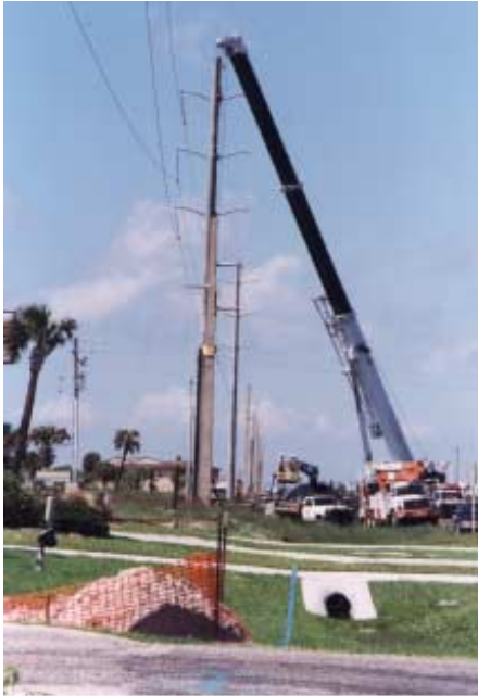
Transmission Line Under Construction
