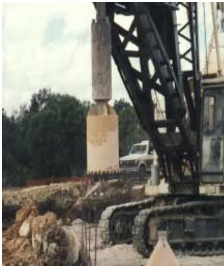
Drilling pier holes for foundations.
